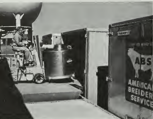
American Breeders Service transports frozen semen to technicians in liquid-nitrogen refrigerators, each with a capacity of 50 thousand ampules. They normally have about 1 million ampules in storage and as many as 50 thousand from one bull.
